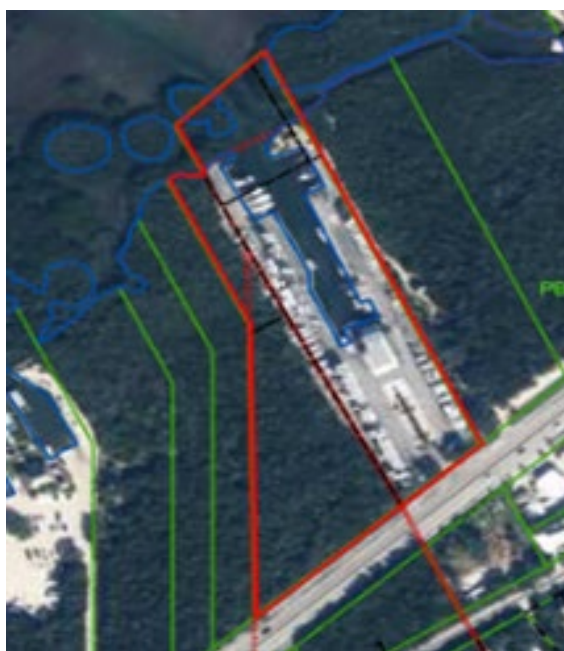
Project Location: 80460 Overseas Hwy – Upper Matecumbe Key
