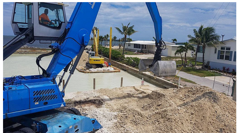
Photo: Canal 25 Backfilling
