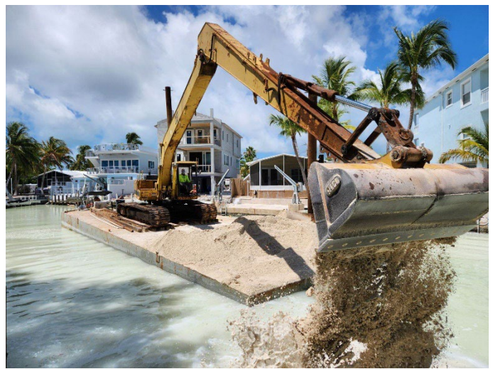
Photo: Canal 90 Backfill Operations
