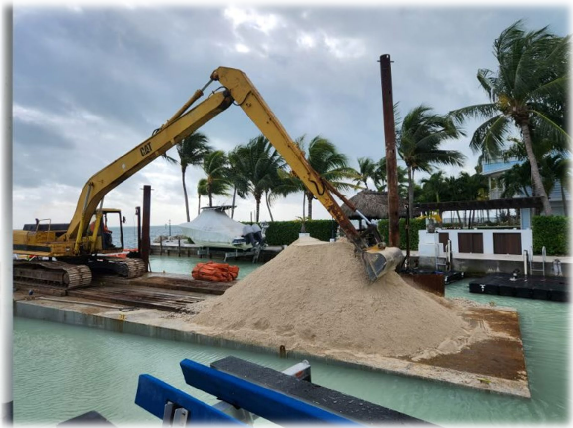
Village of Islamorada Canal #116 In-Progress Photo
