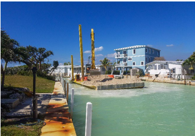
Photo: Canal 28 Backfilling
