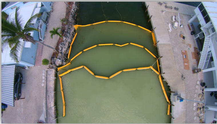
AEI Turbidity System functioning flawlessly at Canal 29 Backfilling project.
