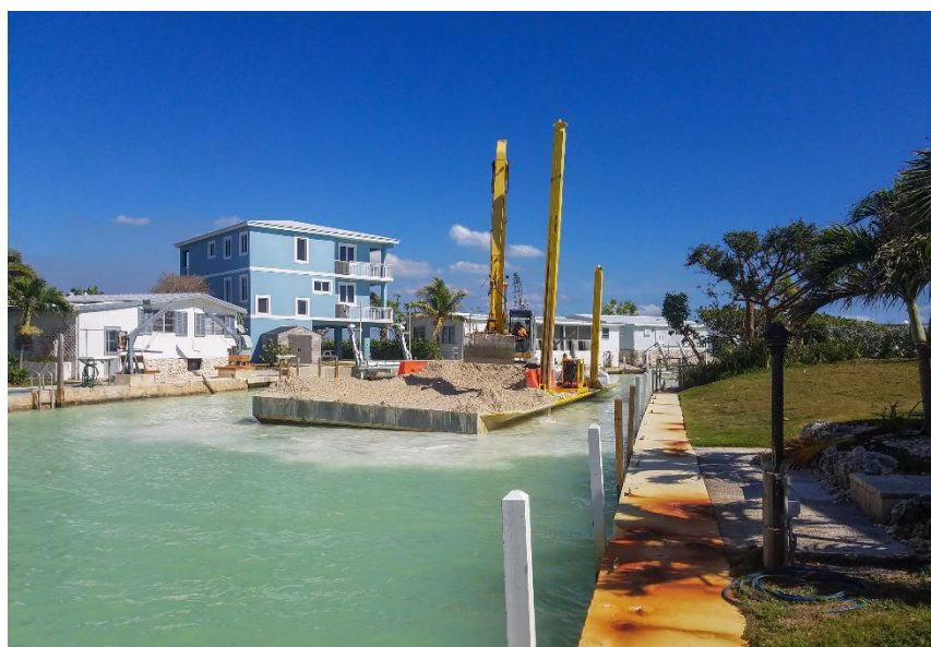
AEI aggregate placement/backfill operations on Canal 25 Water Quality Improvement Project.
