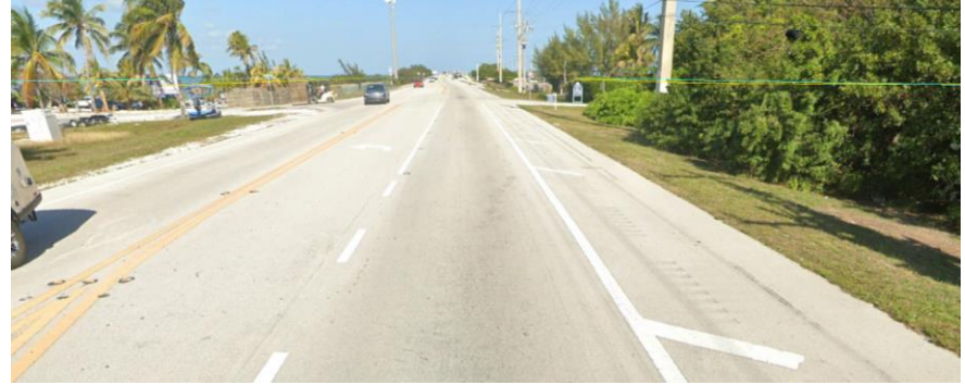
Looking northbound at Conch Avenue
