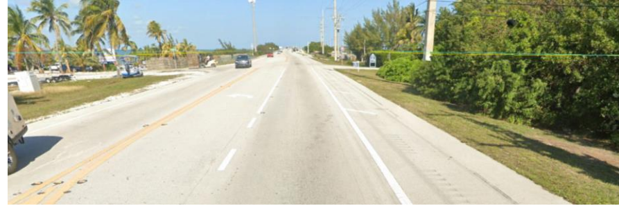
Looking northbound at Conch Avenue
