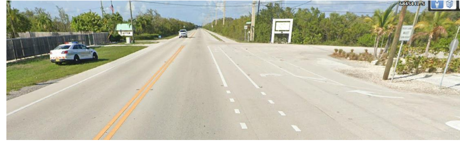
Looking northbound at Layton Drive
