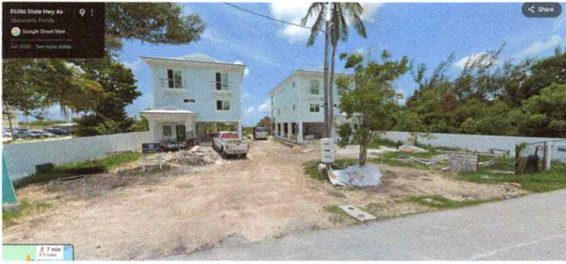
2 houses built after Existing Hog Heaven
